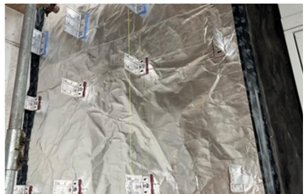
Phase 1 South Elevation
