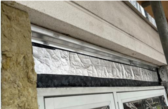
Phase 1 South Elevation
