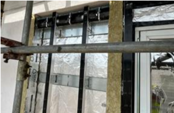
Phase 1 South Elevation
