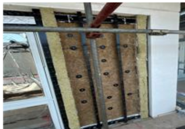
Phase 1 South Elevation
